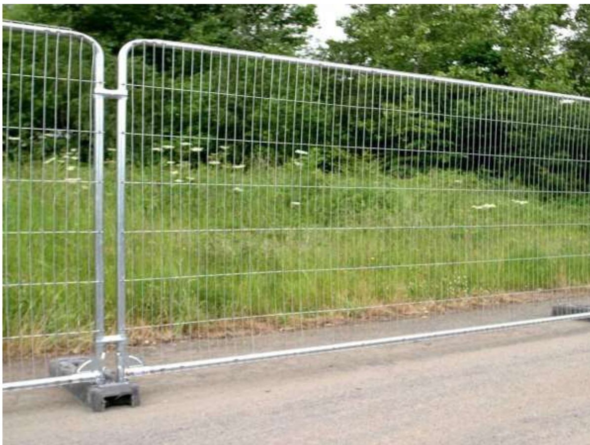
Photo 2 – Typical Heras Type Demountable Fence
