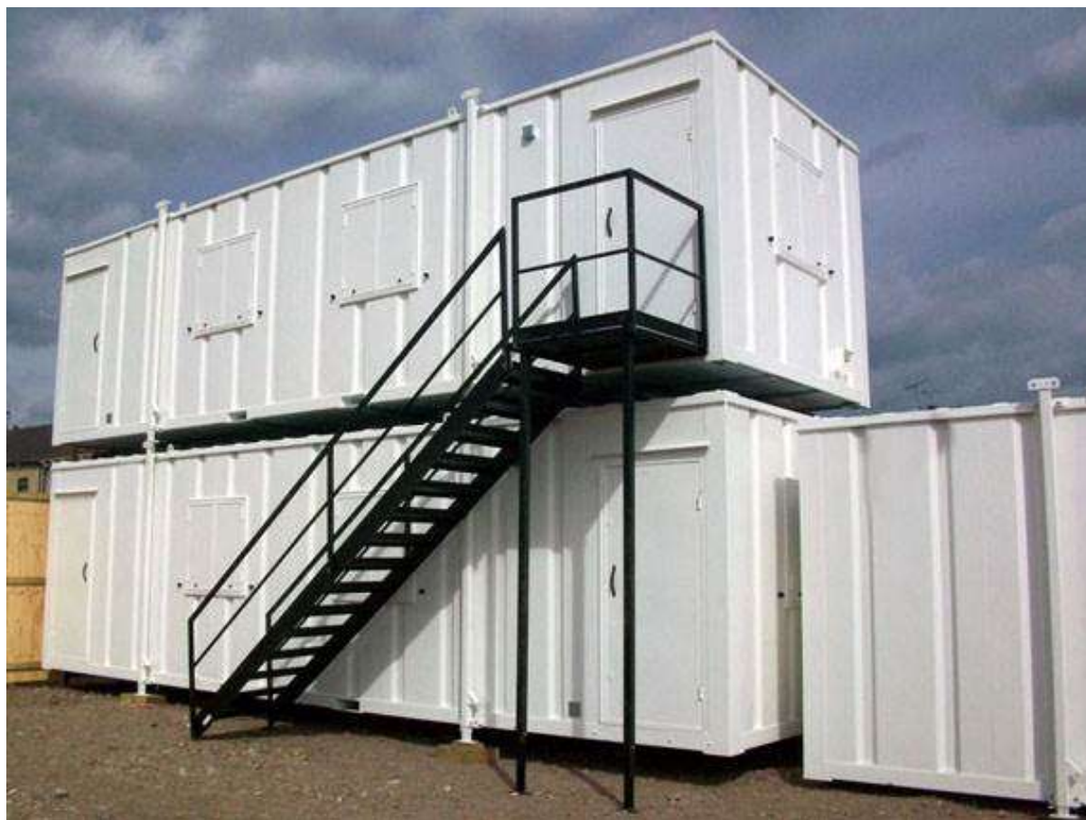
Photo 3 - Typical Stacked Site Containers Where Space is Restricted
