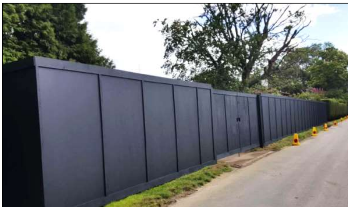
Photo 1 – Typical Site Hoarding Arrangement
